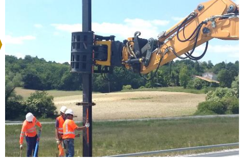
Step 3 Mast Erection & Second Stage Concreting (grouting)
