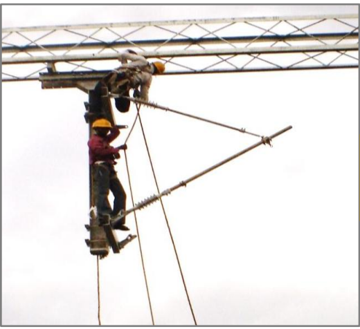
Step 4 Cantilever Erection
