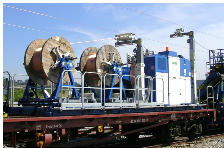
Step 5 Stringing of Conductors using Wiring Train
