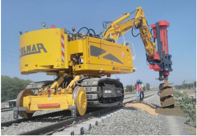
Step 1 Cylindrical Auger Boring
