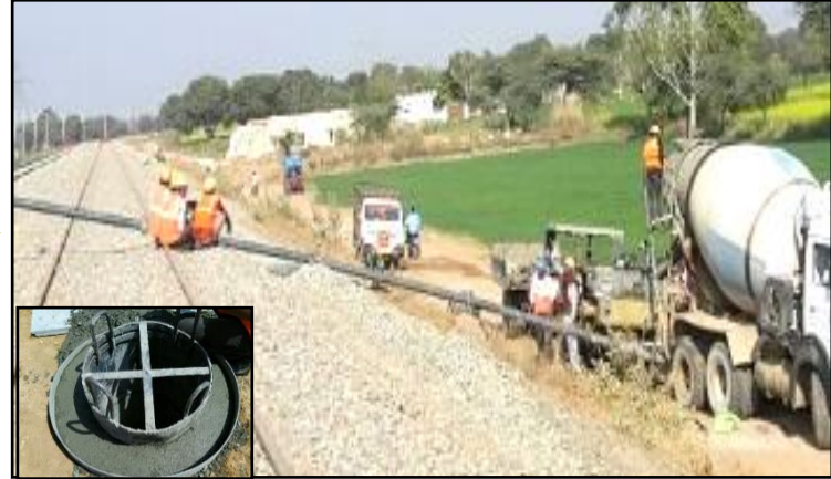
Step 2 1 st Stage - Concreting of Foundation
